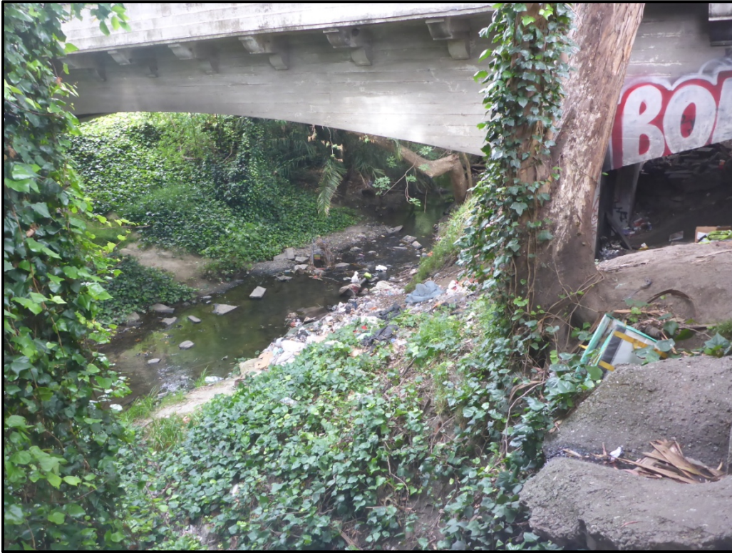
Homeless encampment below bridge located on the western boundary of the Study Area. 2020. Facing southwest.
