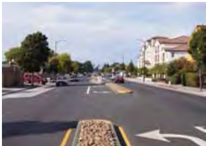
San Pablo Avenue has a diverse array of residential, commercial, and public uses, as well as activity centers that serve as local and regional draws.
