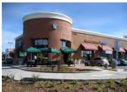
College Center Shops at El Portal Drive.
