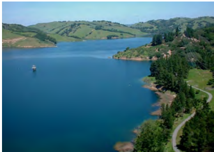
View of San Pablo Reservoir
